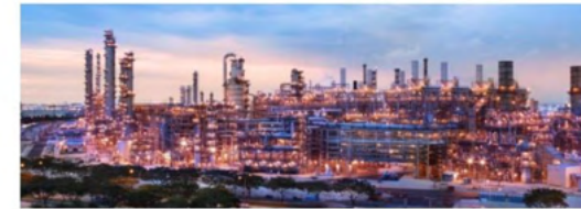
A large petrochemical plant
