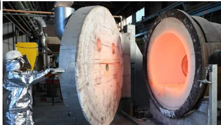
2 MW Pilot reheat / heat-treat furnace
